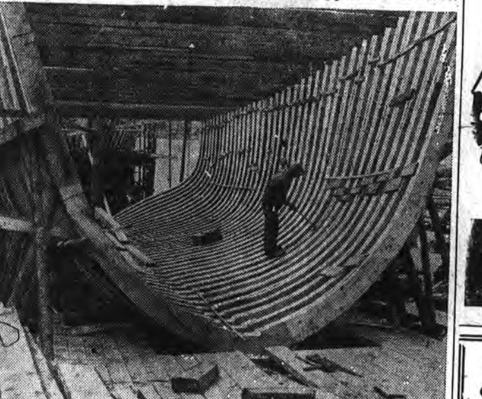
Old-timer Ray Rubshaw is working inside the framework of a hull under construction. He is dubbing or smoothing out and lining up the ribs for planking, using an axe.
